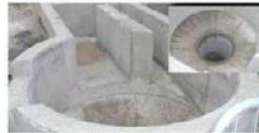
Civil construction and installation.
