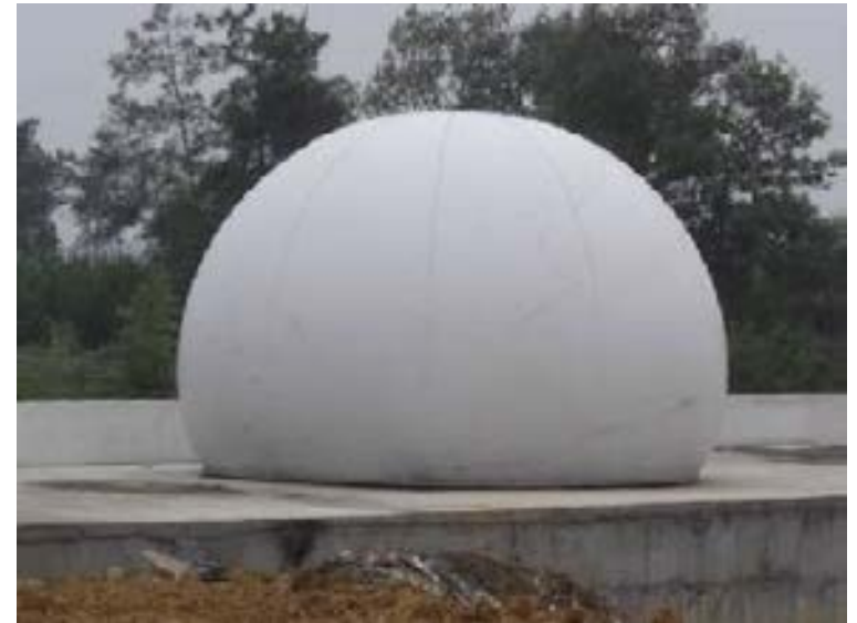
Biogas Storage Dome
