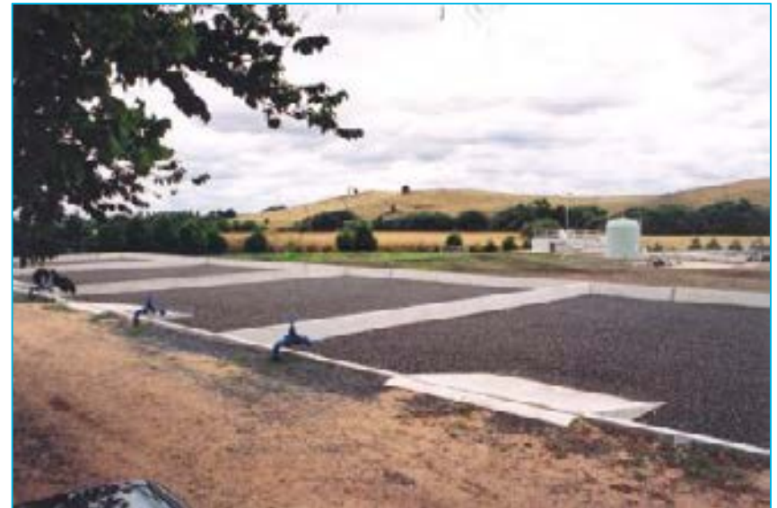
Sand Bed Drying
