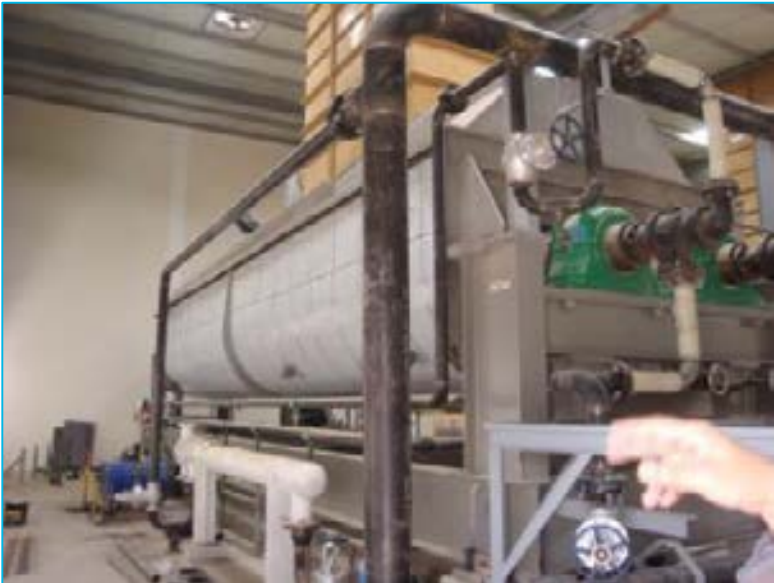
In-vessel Thermal Drying
